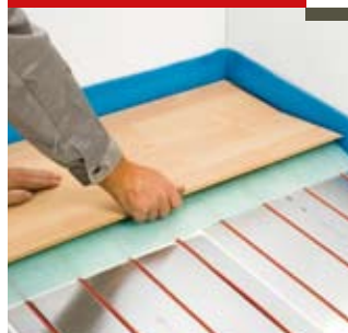
Installation of the wooden floor
